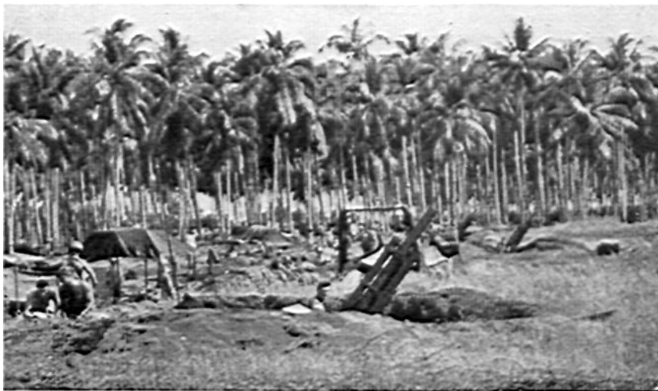
A 105 battery dug in on Guadalcanal
